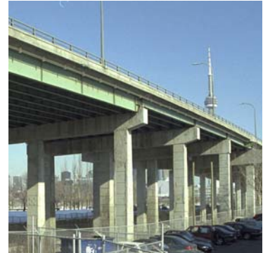
View of the existing Gardiner Expressway, looking toward the Fort from Garrison Road, north of the Fort York Armouries.
