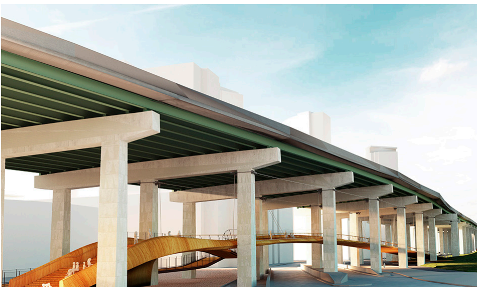
The project hopes to create a suspended timber bridge to provide a safe crossing at Fort York Boulevard. A key feature in the bridge's design is a rolled timber bench running along its south edge. The bridge and the seating will provide a new panoramic view of the Fort York National Historic Site's lawns and buildings. (Image courtesy of PUBLIC WORK)
