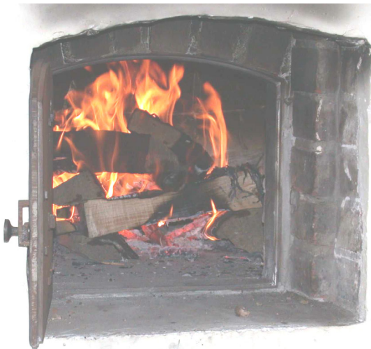
The first firing of the newly restored brick bake oven.
