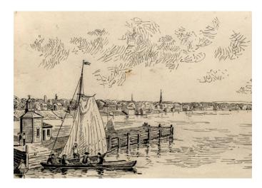
**The Queen's Wharf** at the foot of Bathurst, looking toward Toronto harbour. This is part of a pen-and-ink drawing done by Owen Staples after an 1847 lithograph. It shows the crib construction of the wharf and the original lighthouse built in 1838, the year after the wharf was extended to the point seen here. Courtesy Toronto Public Library (Baldwin B 1-9b)
