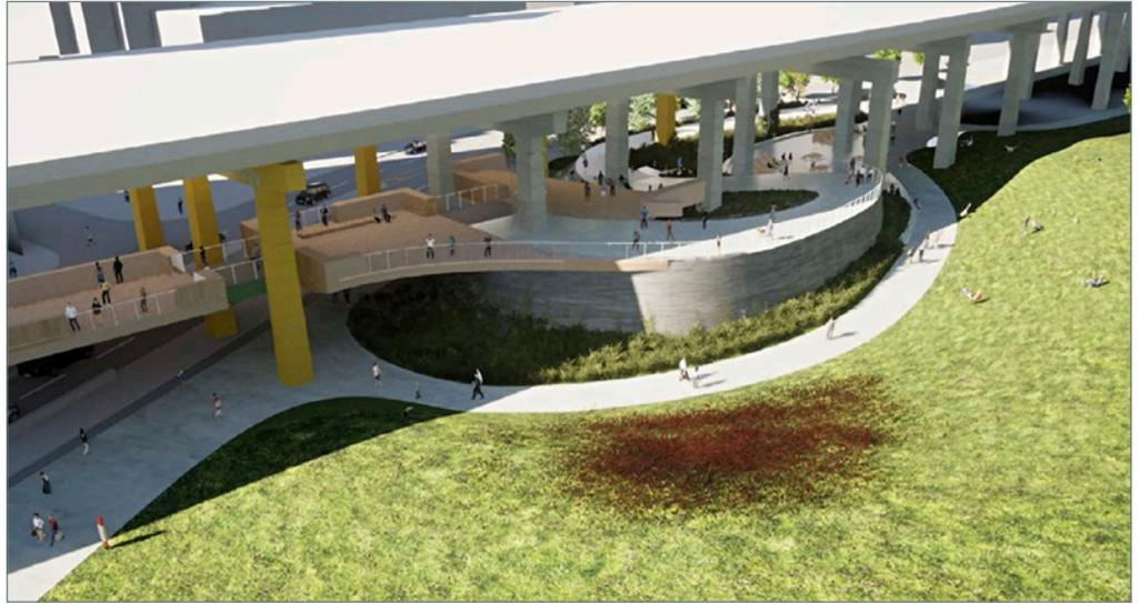
**Drones-eye view of the West Landing** The decks and the curving ramp are higher than the fort's southern rampart, and the massive masonry wall sits on the old Lake Ontario shoreline. The red blotch in the foreground represents the Magazine Crater, while Fort York Blvd can be seen in the distance beneath the Gardiner Expressway. Rendering by Public Work
